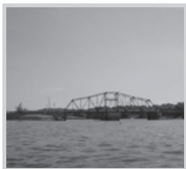
Photo: Historic Berkley-Dighton Bridge.
