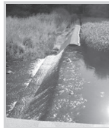
Photo: Segreganset River Dam, Dighton.
